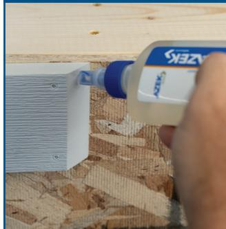
Use AZEK adhesive at trim joints to minimize gaps from expansion and contraction.
